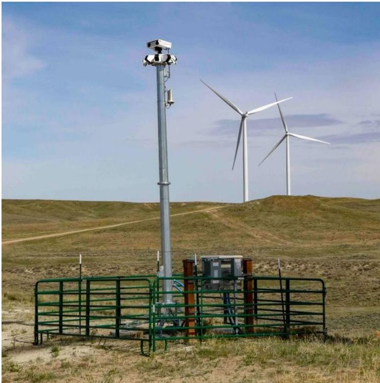
Duke Energy began installing sky-scanning IdentiFlight robots at a Wyoming wind farm in 2015. A study said the technology has helped reduce bird deaths. PHOTO: IDENTIFLIGHT
